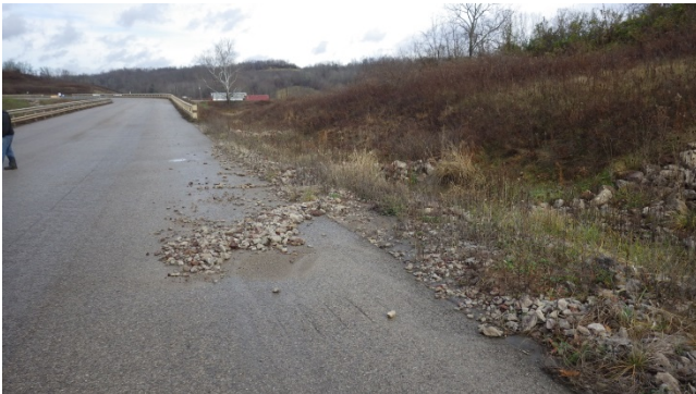
Photo 29 Washout of riprap-lined surface water channel on east side of the perimeter road east of Sediment Trap No. 26.
