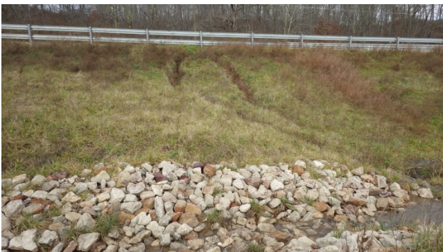
Photo 30 Erosion gullies approximately 24 inches deep were observed on the south side of the perimeter road near the northeast corner of the East Sedimentation Pond.
